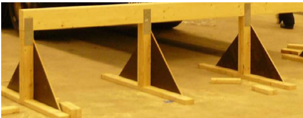
Figure 6. Floor element supporting glulam beam, studs and stabilizing plywood slabs.
