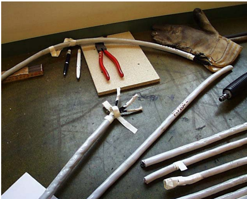
Figure A2-4. Insulating tape applied on cable.
