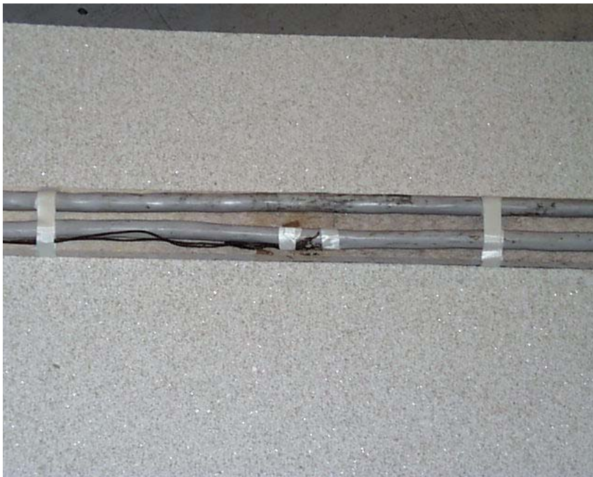
Figure A2-6. A closer look at the thermocouple mounting.
