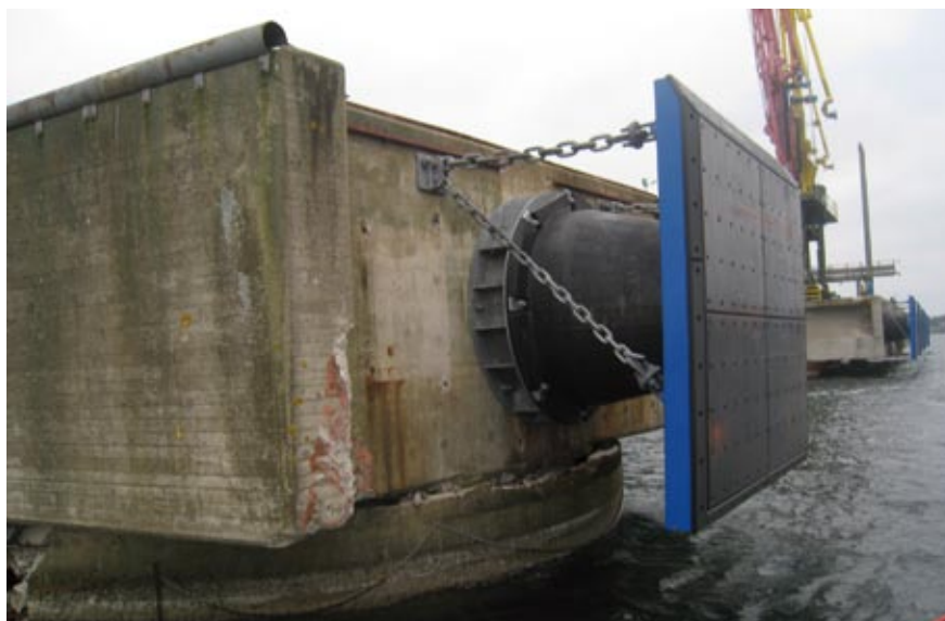
Figur 2. Skadad dykdalb.
