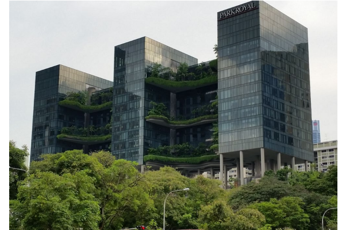
"Green" Building in Singapore, Courtesy Brian Meacham.
