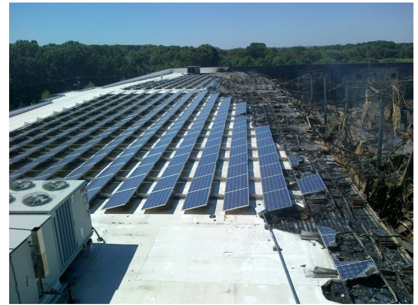
Figure 3.9 Aftermath of Delanco, NJ, Warehouse Fire (Courtesy of New Jersey State Fire Marshal Office)
