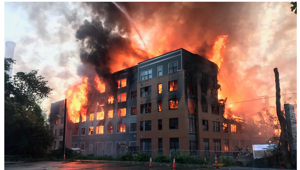
Figure 3.10 Fire in Timber Frame Apartment Building Under Construction (Source: Captain John Bonadio, Waltham Fire Department, as published at https://www.enr.com/articles/42484-what-local-officials-want-to-do-about-wood-frame-building-fires-in-massachusetts ), Courtesy of Waltham, Massachusetts Fire Department)
