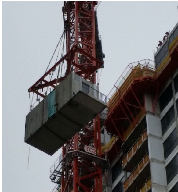
Modular Construction in Singapore, Courtesy Brian Meacham.
