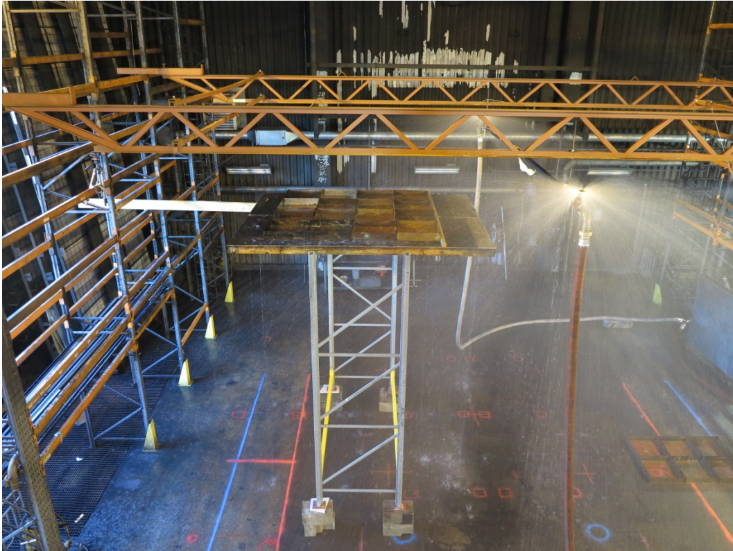
Figure 7 Test 2.5: The water spray pattern of the Tyco model EC-14 sprinkler at a pressure of 0.7 bar and a spacing of 5.0 m. The water flow rate per sprinkler was 162 liter/min.
