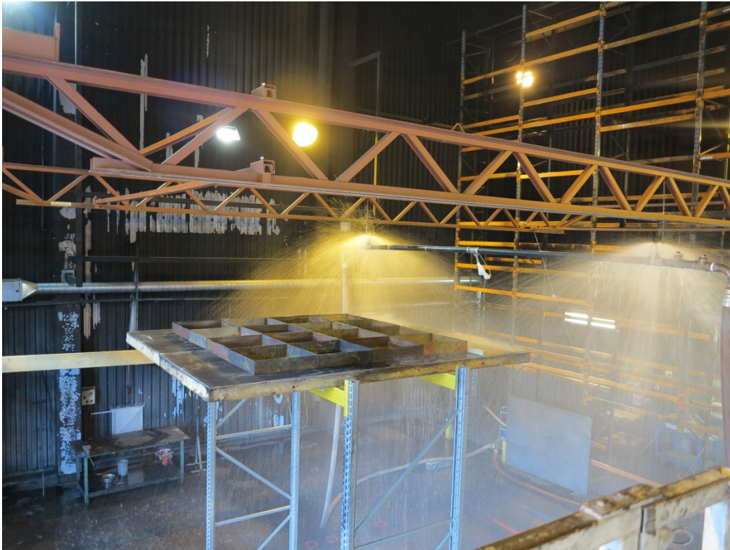
Figure 4 Test 1.2: The water spray pattern of the Tyco model EC-25 sprinkler at a pressure of 0.56 bar and a spacing of 4.2 m. The water flow rate per sprinkler was 266 liter/min.
