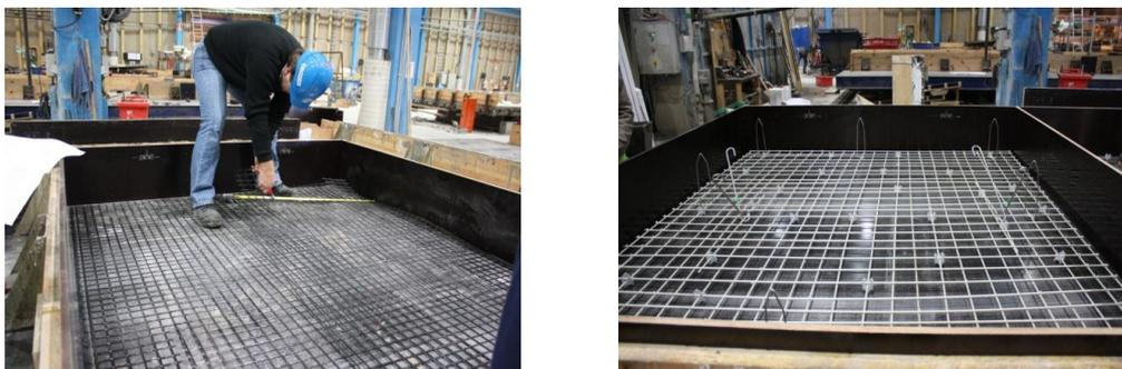
*Figure 3 – Preparation of the reinforcement (carbon fiber –left; glass fiber –right)*
