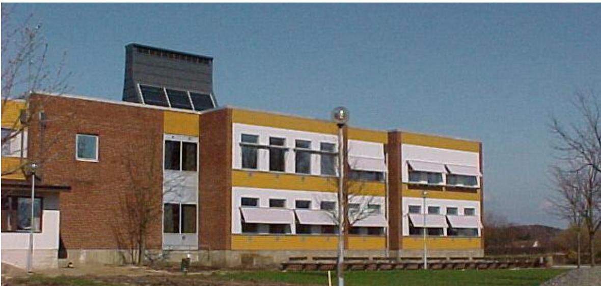
**Figure 1. Picture of the Tånga School. Supply air intakes are placed below the windows. The right half shows one wing of the building with the solar chimney on the roof.**
