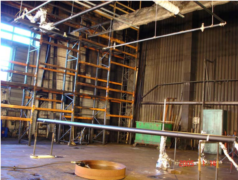
Figure 5 The smallest of the fire trays. Note the Pipe Thermometer directly above the fire tray and the Pipe Thermometer above the water spray system grid.
