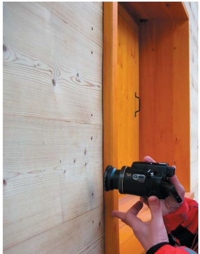
*Close inspection of heat treated spruce cladding.*
