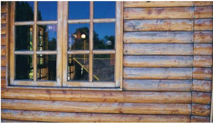
Clear-coated cladding with severe UV degradation and flaking lacquer.
