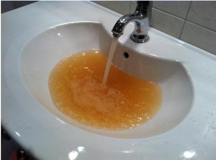
**Figure 3 – Discolored drinking water is the most common problem caused by direct connection of fire sprinkler systems to the water mains.**
