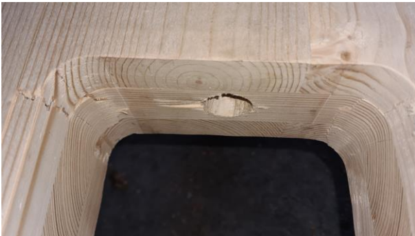
Figure 17: Test 3 local damage under the washer
