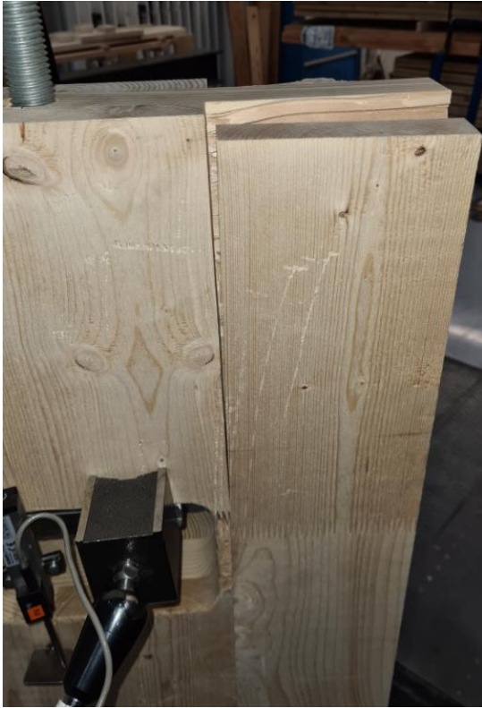
Figure 16: Test 3 shear and finger joint failure
