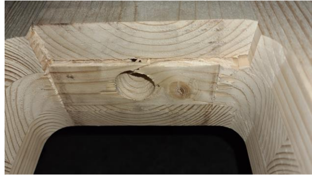
Figure 14: Test 2 local failure under the washer
