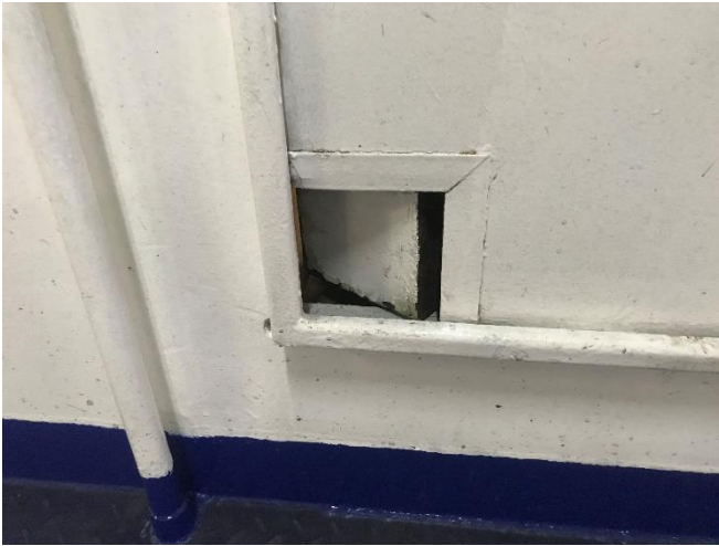
Figure 6 Example of “cat hole” in hinged door
