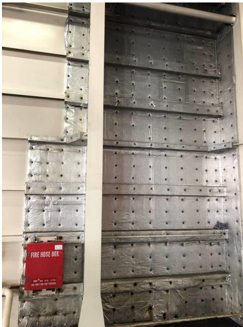
Figure 5 Example of undamaged insulation
