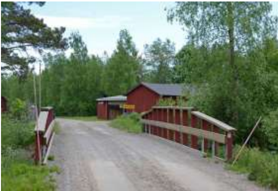
A typical Swedish Road Bridge built with a stressed laminated glulam deck made of spruce.
