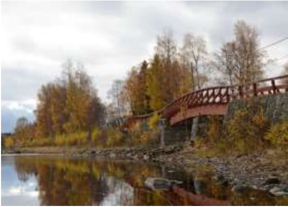
Three small Road Bridges over Sävarån.
