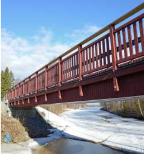
Pedestrian Bridge with box-beam deck.
