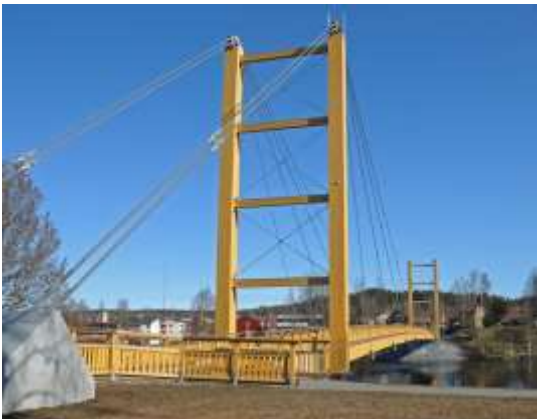
Pedestrian bridge over Skellefteälven. The estimated service life is 80 years.
