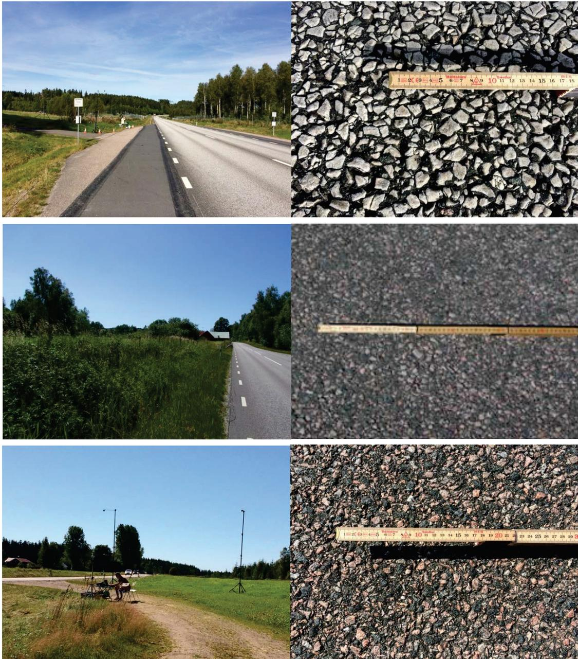
Figure 2 Three examples of measurement sites and road surfaces (SMA 0/16)
