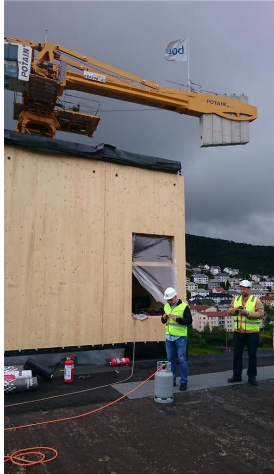
**Figure 15:** Fire extinguishing devices are required for the works with high temperatures.
