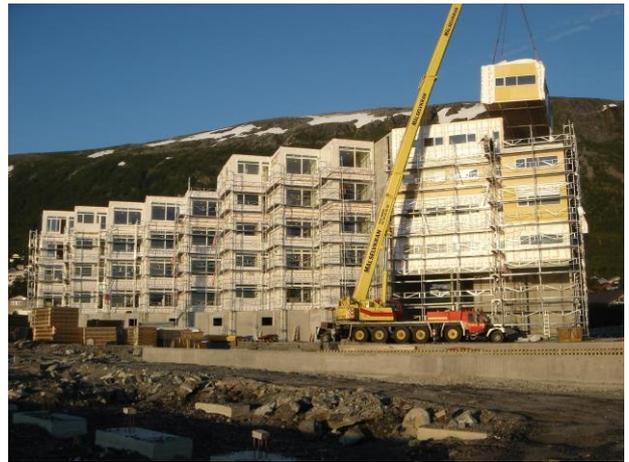
**Figure 8:** *Execution of module houses.*
