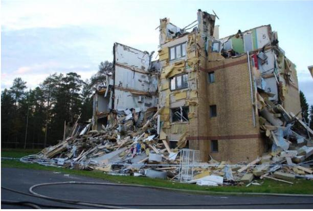
**Figure 10:** Fire spread through the cavities between the timber modules. Fire in Luleå 2013.
