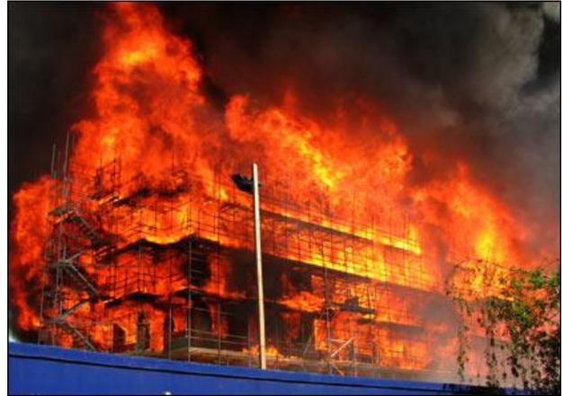
**Figure 4:** Fire in timber frame building occurred during the execution. Colindale. July 2006. Photo: Wei Yecheng
