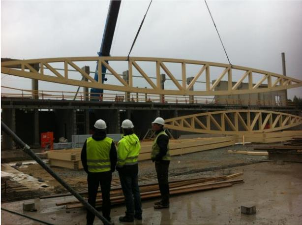
**Figure 3:** Execution of glulam roof trusses.
