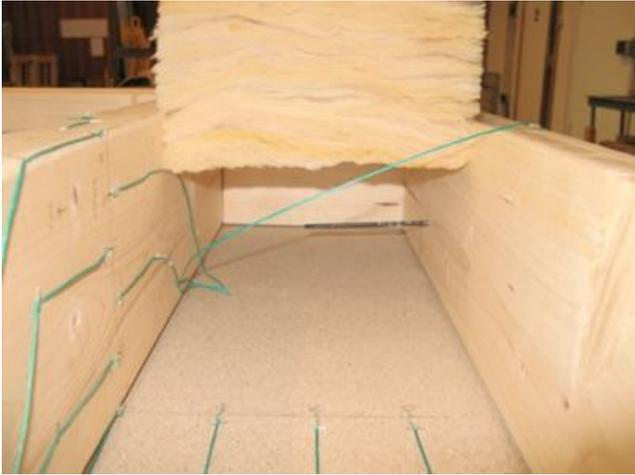
**Figure 14:** Fixing of insulation material by overdimensioning.
