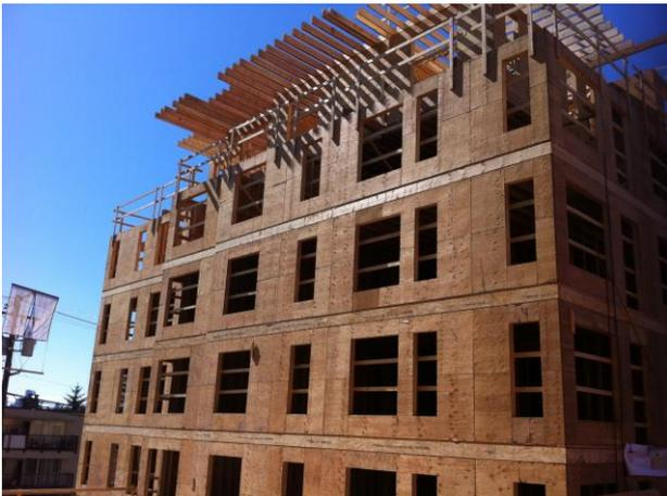
**Figure 6:** *Timber buildings with large amounts of unprotected timber at the execution phase can be sensitive for the fire risk.*
